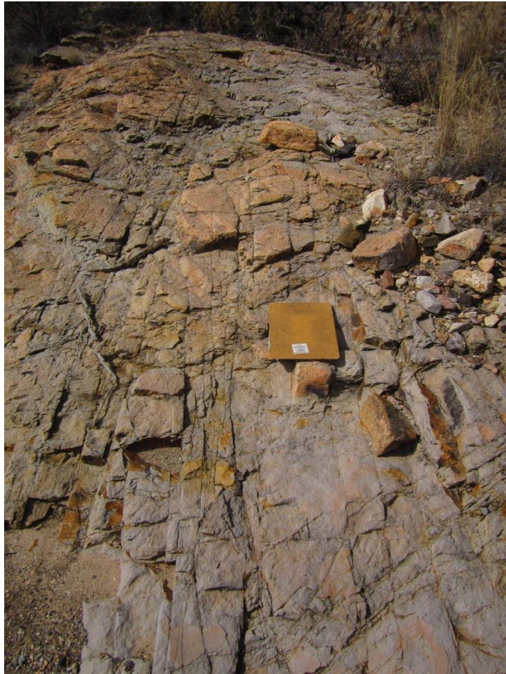
Figure 1.1: Vertical, aligned cracks, fractures, and subsurface stress regimes are common causes of azimuthal anisotropy.
