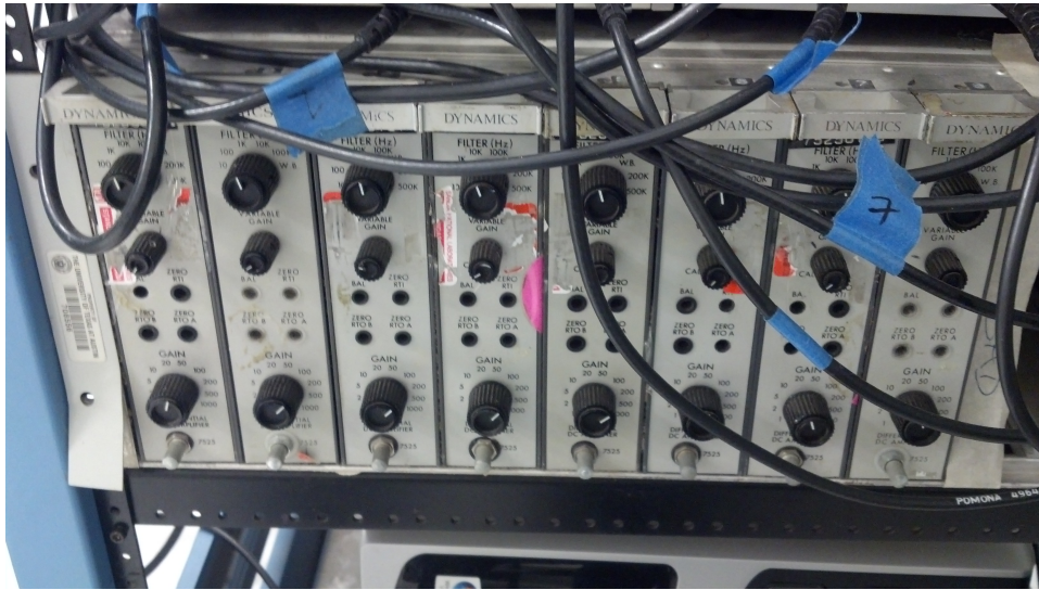
Figure 3.2: Electrical Amplifiers for Kulite Transducers
