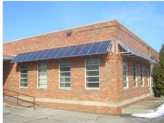
Fig A.10 Doty and Miller Office, courtesy of National Park Service
