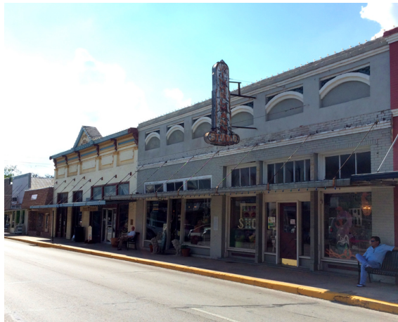
Figure 30: North side of West Alamo Street
