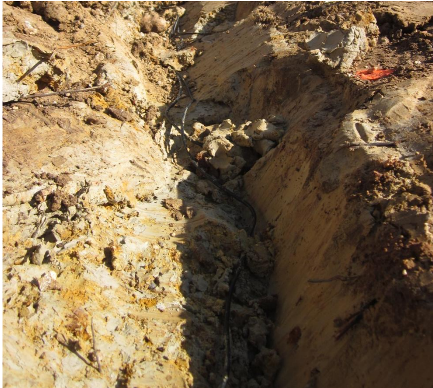
Figure 3.2: Exposed Cut of Cook Mountain Formation during Installation of Moisture Sensors
