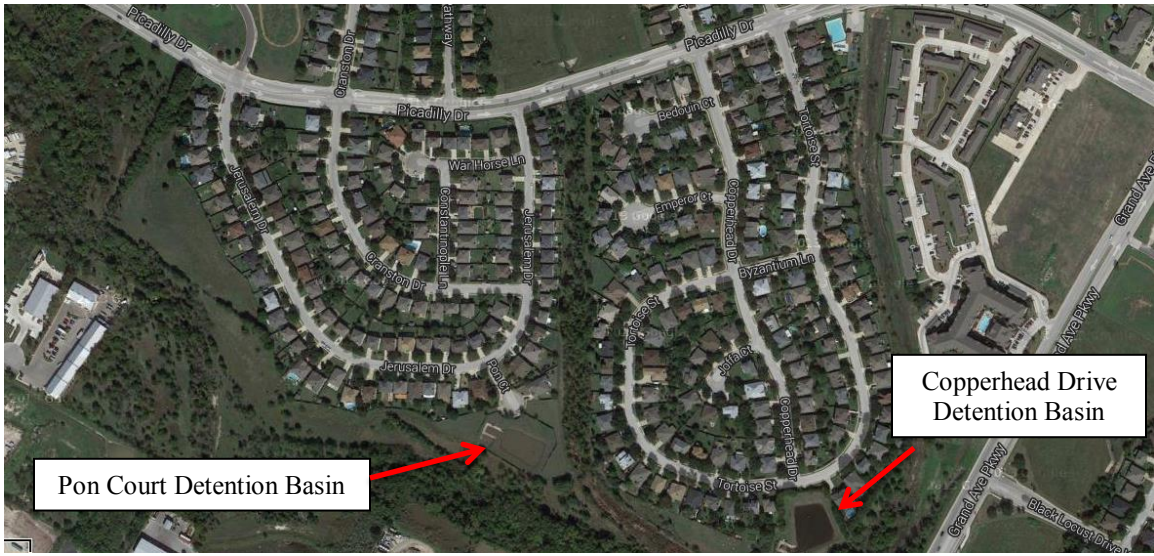
Figure 1. Location of Pon Court and Copperhead Drive Stormwater Detention Basins in Pflugerville, Texas (Google Maps, 2014).
