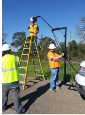
Figure 3.37: Installing the digital camera on the mounting system
