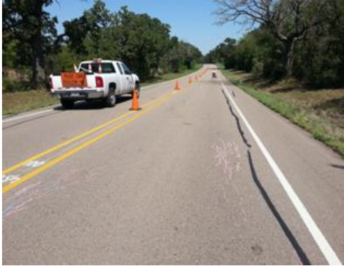
Figure 3.36: Traffic control, pilot car, and flaggers
