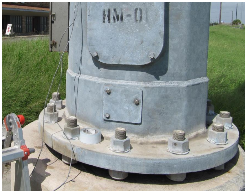
Figure 1.2: Typical base plate connection
