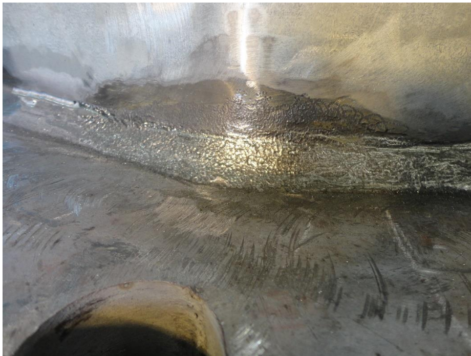
Figure A.4: Final result after repair
