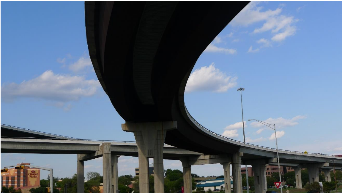
Figure 1.1: High Mast Illumination Pole in service at highway intersection
