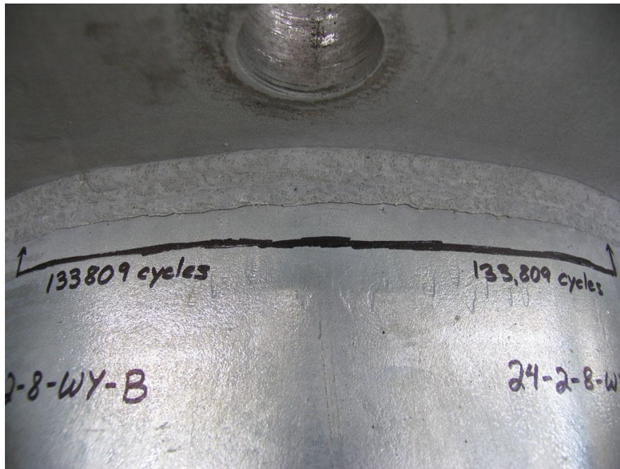
Figure 2.16: Typical failure of Wyoming full penetration weld connection (Rios, 2007)
