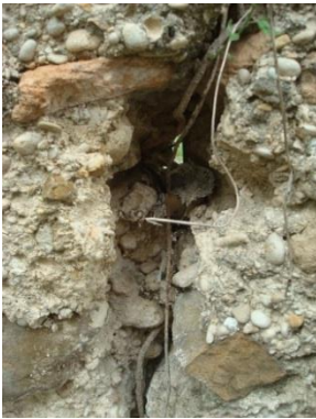
Figure 4.5: Riverside Cemetery Wall, Author's image, September 19, 2013. This image shows the areas where two wall sections are joined. Samples were extracted just to the outside of this joint.
