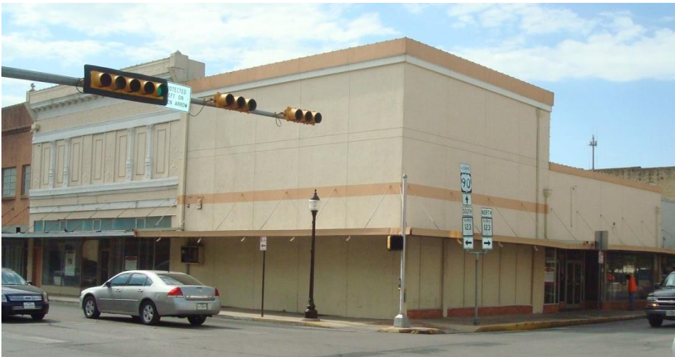
Figure 2.4: Moses Campbell Commercial Building, Author's image, May 1, 2014. The photo was taken from the southeast corner of the E. Court St. and N. Austin St. intersection. The Moses Campbell Commercial Building is the corner structure. The adjoining buildings to the west and to the north were renovated in the mid to late 20 th century to join the Moses Campbell building. The concrete wall is located between the Campbell building and the building to the north.
