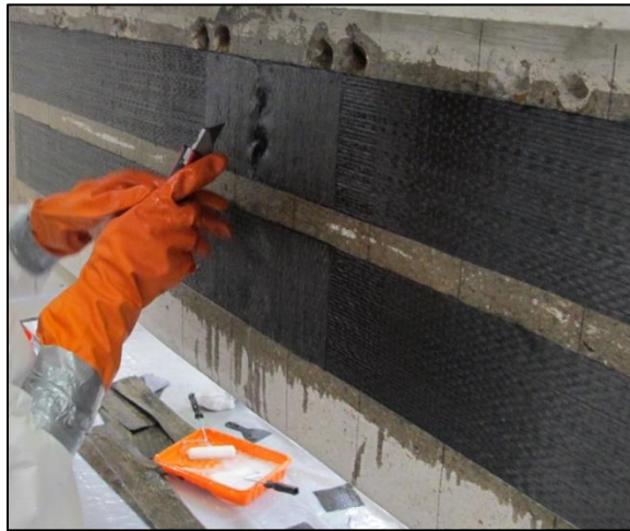
Figure 3-54 Making an opening for the anchor using a knife
