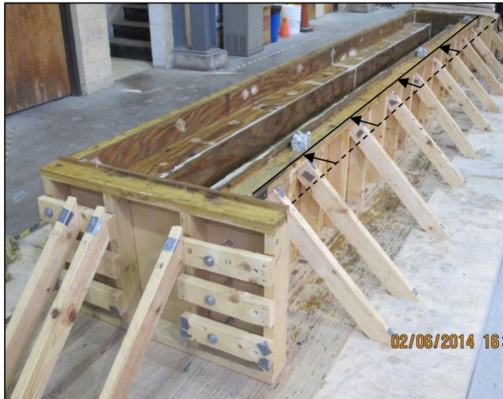
Figure 3-12: Formwork for 8-in. web specimen by shifting one side
