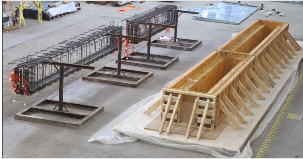
Figure 3-20: Steel cages and formwork before placement for 14-in. specimen
