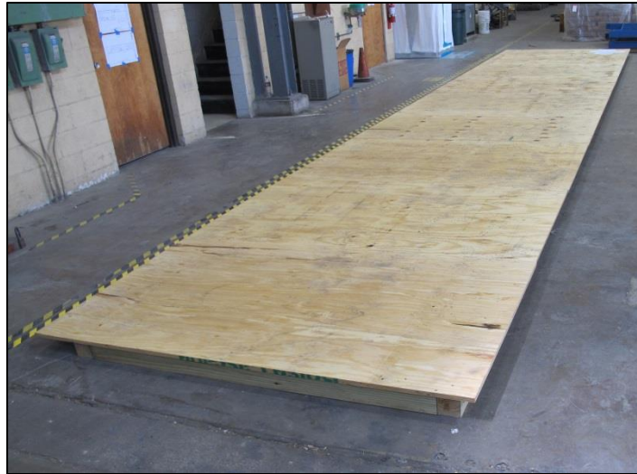
Figure 3-7: Formwork's strong base
