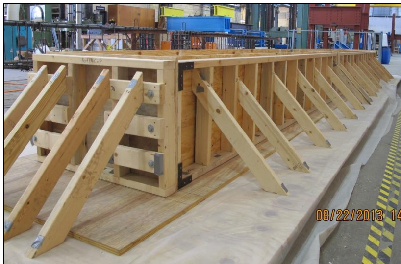
Figure 3-11: 2x4 kickers for lateral support
