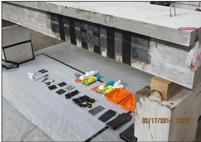
Figure 3-43: Preparation for CFRP installation
