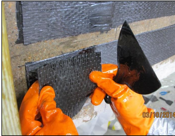
Figure 3-53: First 5x5-in patch placed on top of the hole location
