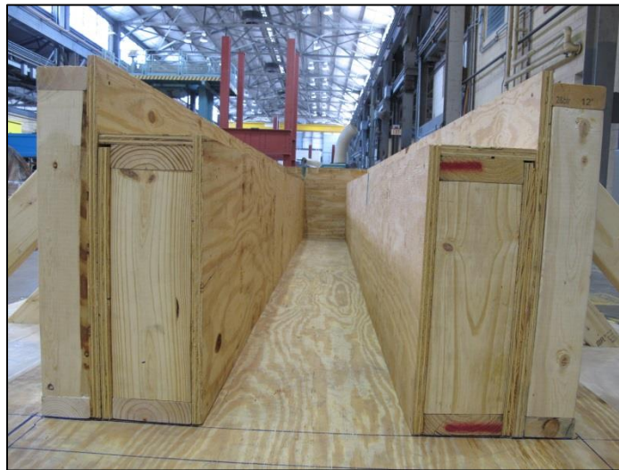
Figure 3-8: As-built formwork for 14-in. specimen
