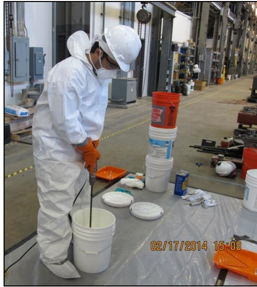
Figure 3-46: Mixing epoxy components
