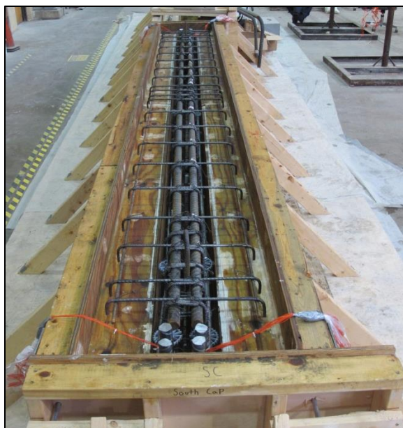
Figure 3-22: Placement of steel cage in the formwork for 8-in. specimen
