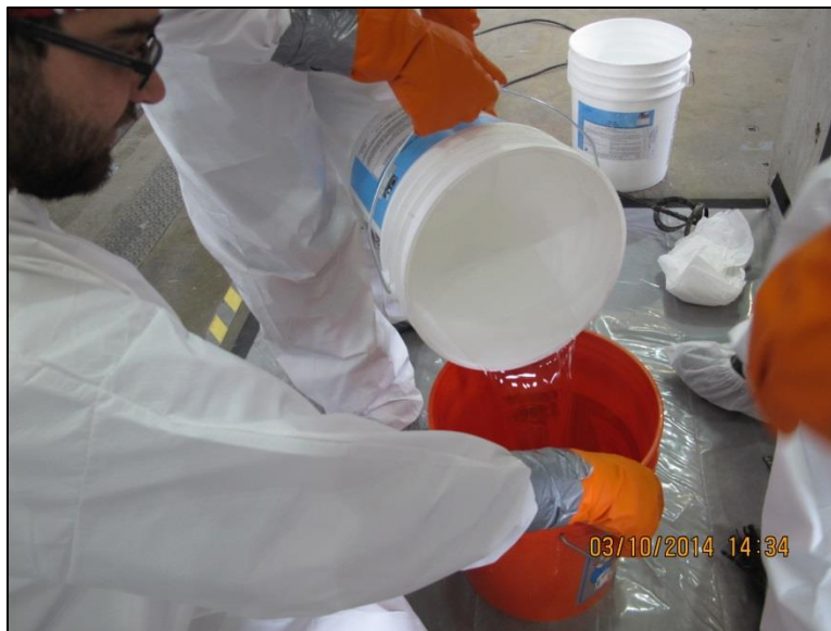
Figure 3-45: Proportioning the epoxy components
