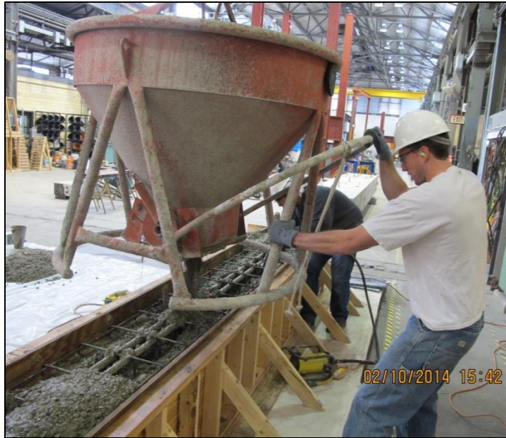
Figure 3-23: Concrete placement using one cubic yard concrete bucket
