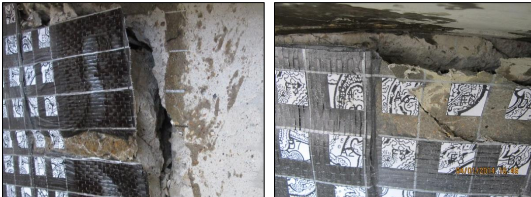
Figure 4-98: Failure mode of 8-3-Bi-D due to extreme loading
