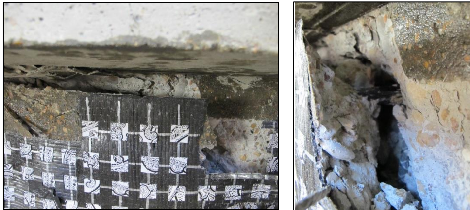
Figure 4-19: Separation of CFRP strip and anchor as one unit
