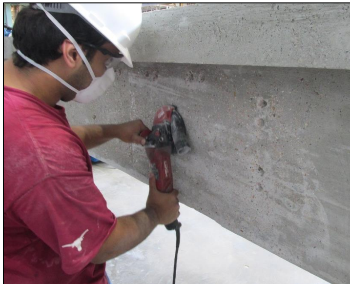
Figure 3-30: Grinding the concrete surface to apply CFRP laminates
