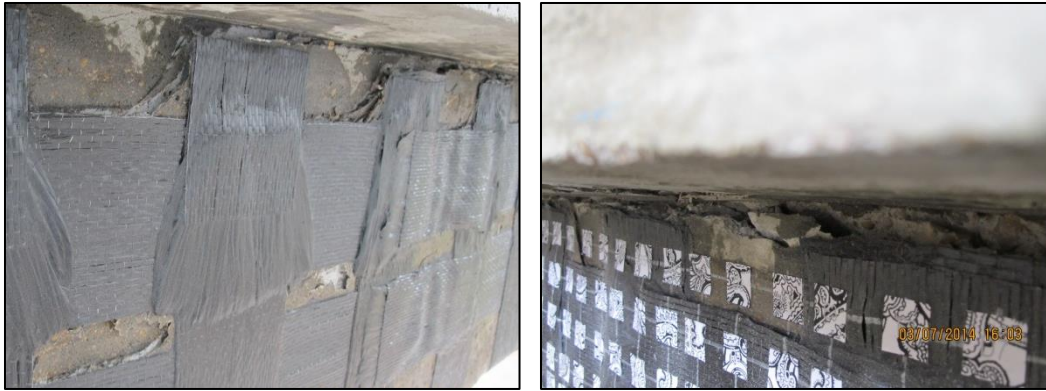
Figure 4-45: Separation of CFRP strips
