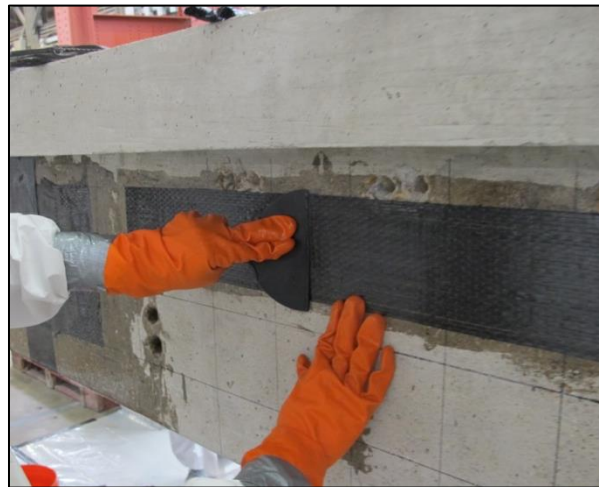
Figure 3-52: Removing excessive epoxy from the strip using plastic putty knife
