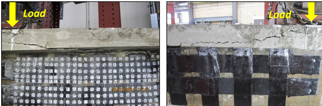
Figure 4-44: Critical crack in 14-3-Bi-D: left (east), right (west)
