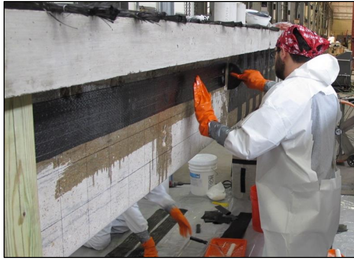
Figure 3-51: Attaching horizontal CFRP strip
