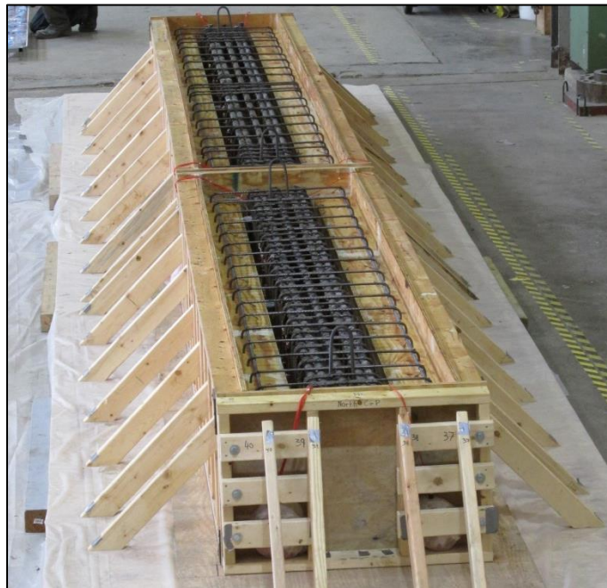
Figure 3-21: Placement of steel cages in the formwork for 14-in. specimens
