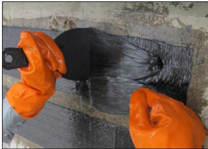
Figure 3-55: Removing excessive epoxy from CFRP anchor
