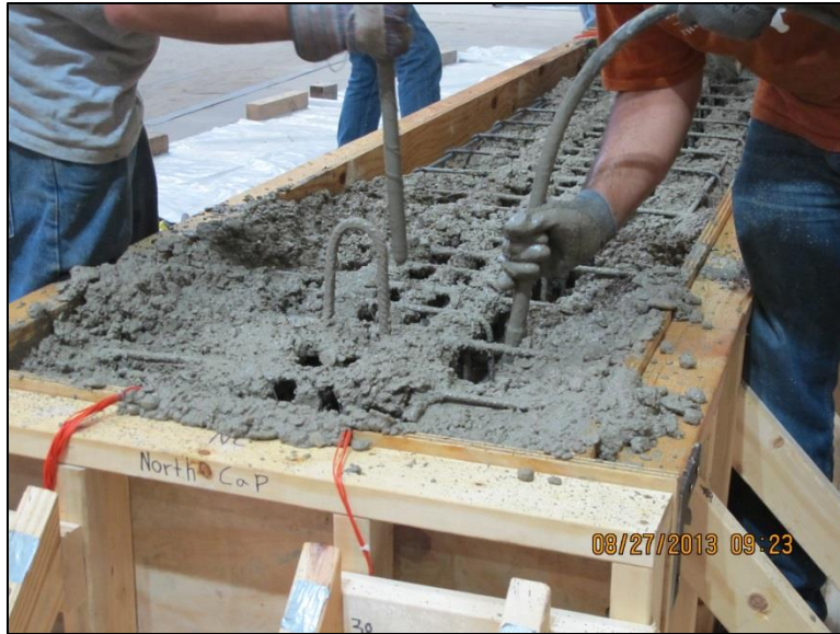
Figure 3-24: Vibrating the concrete by electrical vibrators
