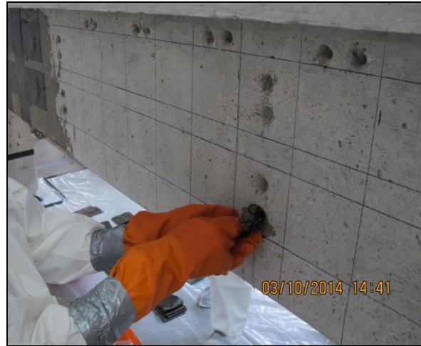
Figure 3-48: Saturating anchor holes using bundled CFRP strip
