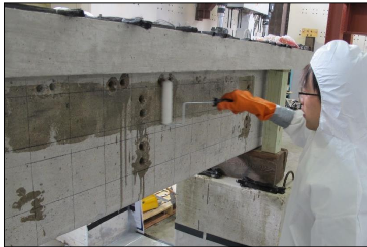
Figure 3-49: Saturating the concrete surface before CFRP application
