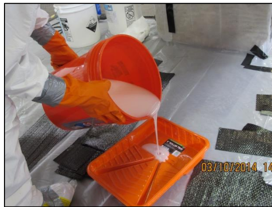
Figure 3-47: Pouring the epoxy in small trays
