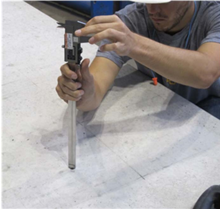
Figure 3-10: Confirming Hole Depth using Digital Calipers for Installation of Wedge Anchor
