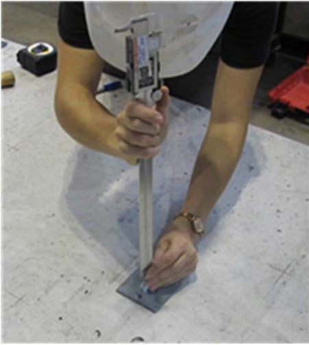
Figure 3-14: Confirming Proper Embedment Depth of Wedge Anchor
