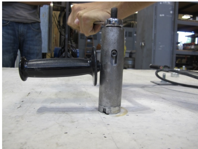
Figure 3-16: Using Setting Tool to Set Undercut Anchor
