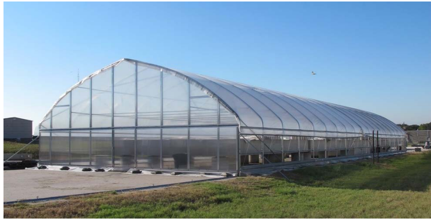
Figure 3-5: Environmental Conditioning Facility with Open Sidewalls
