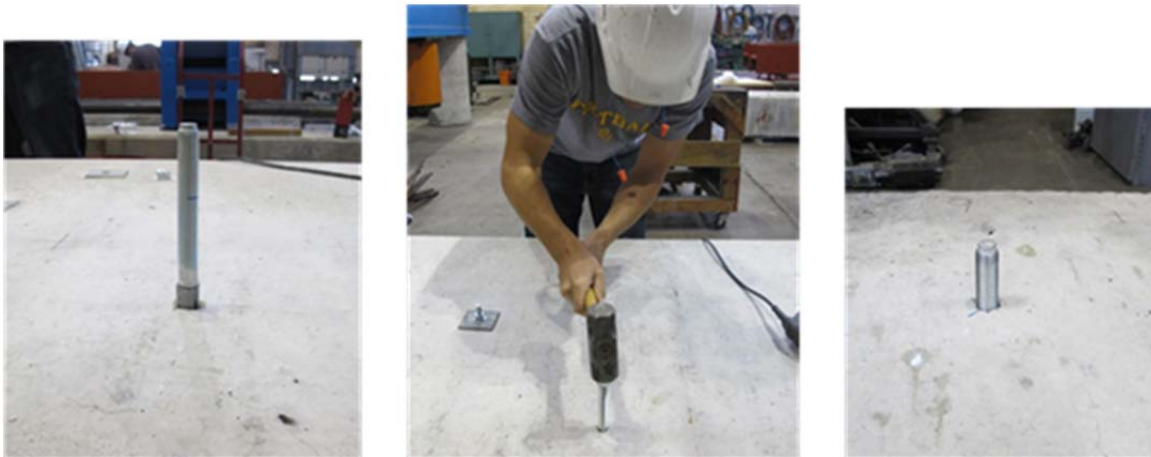
Figure 3-11: Inserting Wedge Anchor into Hole
