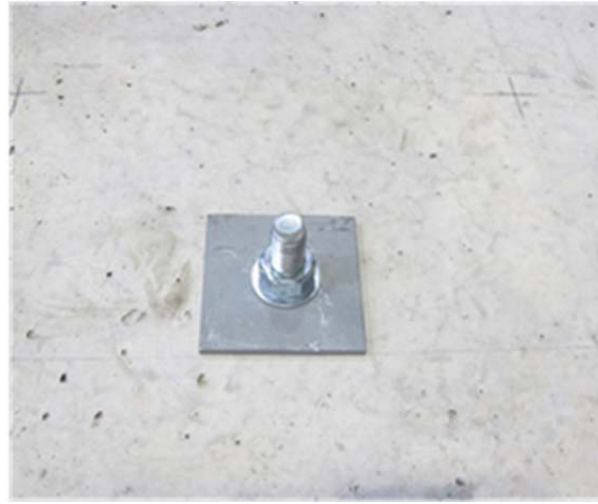
Figure 3-14: Confirming Proper Embedment Depth of Wedge Anchor
