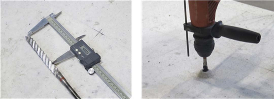
Figure 3-9: Setting Drill Depth and Drilling Hole for Installation of Wedge Anchor
