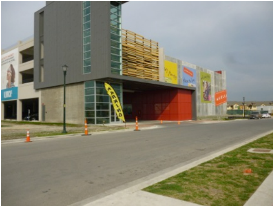
Figure 35: Entrance to shared parking garage on McBee Street, just north of the Thinkery.
