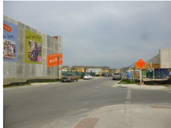
Figure 36: Construction on McBee looking east
