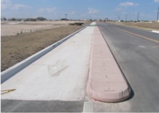
Figure 28: Southbound Cycle Track on Berkman Drive
