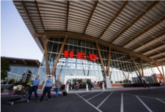
Figure 16: HEB entrance from parking lot
