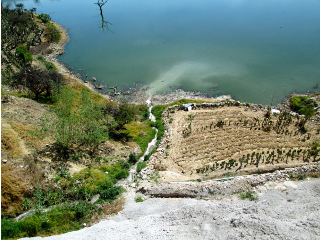
Figure 3: Causes of contamination in the Guadalupe Reservoir include runoff from inadequate wastewater infrastructure (pictured) and illegal dumping of trash.
