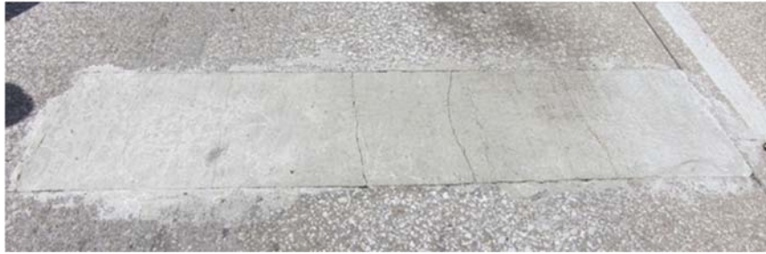
Figure 91: Mixture CSA-2 Repair at Cotulla Site
