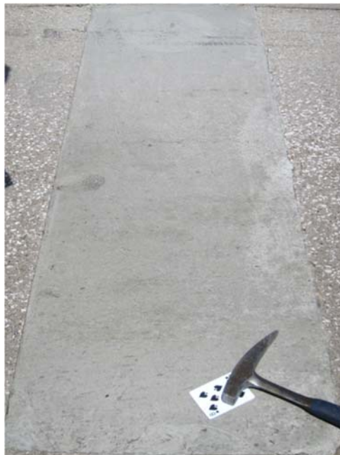
Figure 88: P-2 Mixture Repair at Cotulla Site
