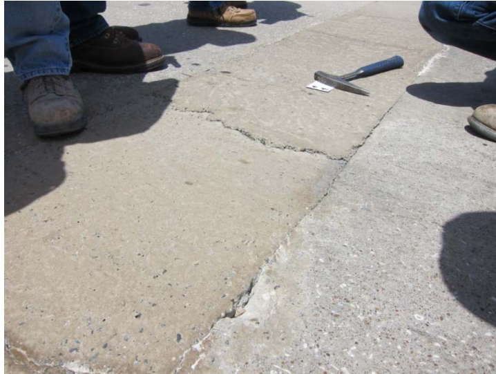
Figure 89: P-AAFA Mixture Repair at Cotulla Site
