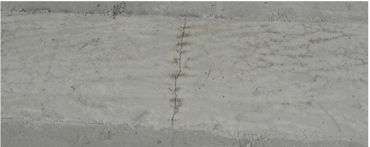
Figure 85: Bridge Deck Repair for CSA-1 Mixture
