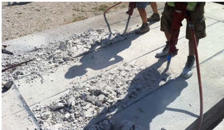
Figure 78: Removal of Existing Concrete using Jackhammers
