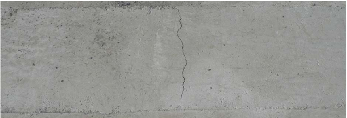
Figure 83: Bridge Deck Repair for PC Type III Mixture
