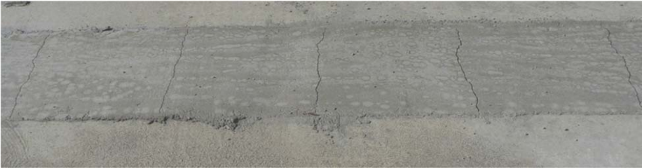
Figure 82: Bridge Deck Repair for CAC-3 Mixture
