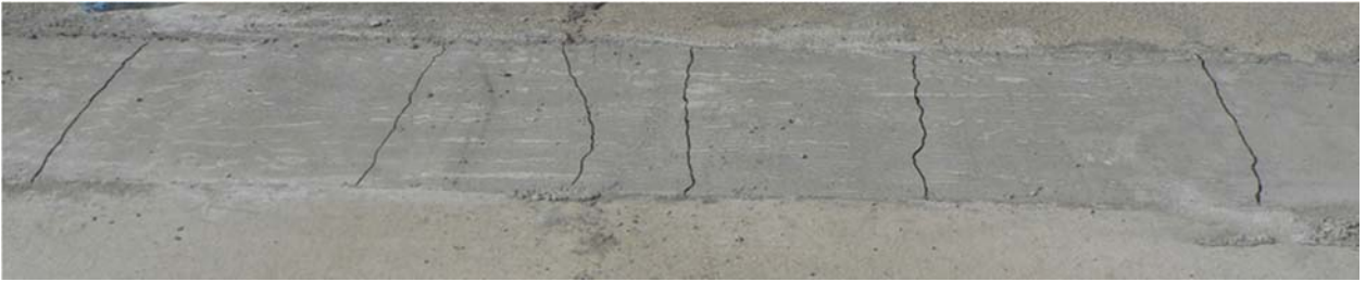
Figure 81: Bridge Deck Repair for P-2 Mixture
