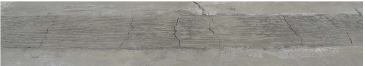
Figure 86: Bridge Deck Repair for CAC-2 Mixture
