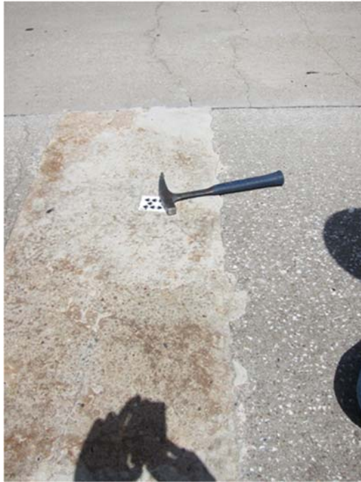
Figure 87: Mixture P-1 Repair at Cotulla Site
