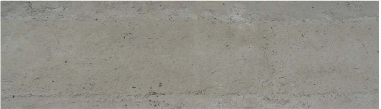
Figure 84: Bridge Deck Repair for P-AAFA Mixture
