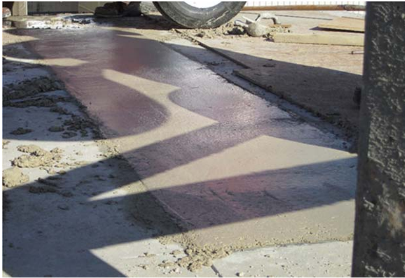
Figure 80: Finished Repair Section before Wet-Cure with Burlap
