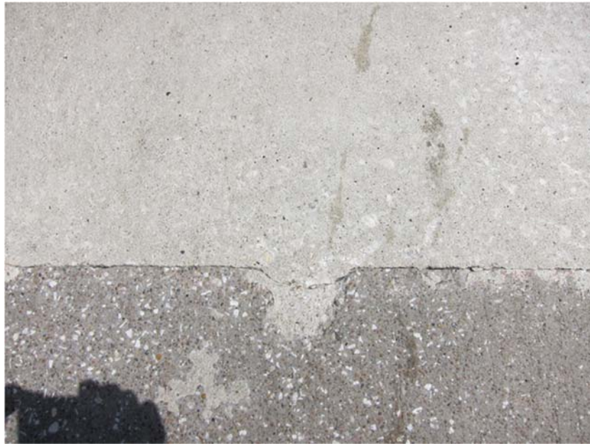
Figure 92: Mixture CSA-3 Bond Interface at Cotulla Site
