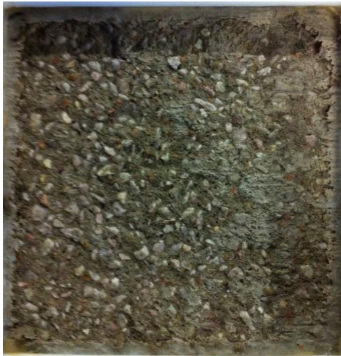
Figure 101. Salt scaling (ASTM C 672) specimen of material CSA-1 after 15 cycles.
