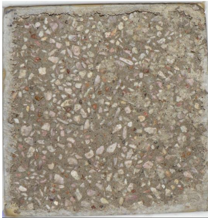
Figure 112. Salt scaling (ASTM C 672) specimen of material CSA-1 after 25 cycles.
