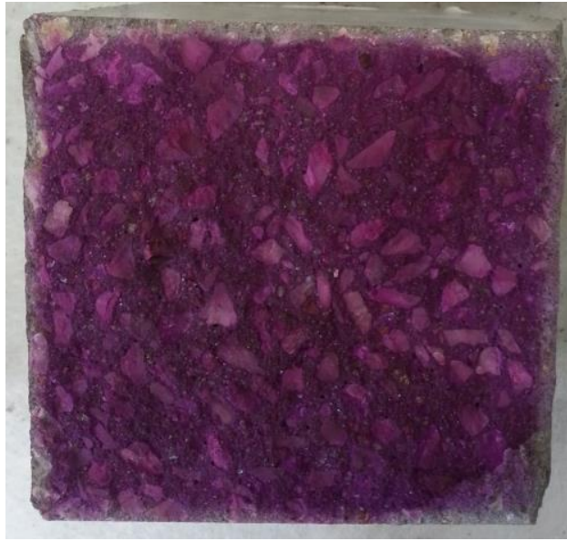
Figure 45. P-2 sample displaying carbonation depth at 11 months using Phenolphthalein PH indicator.
