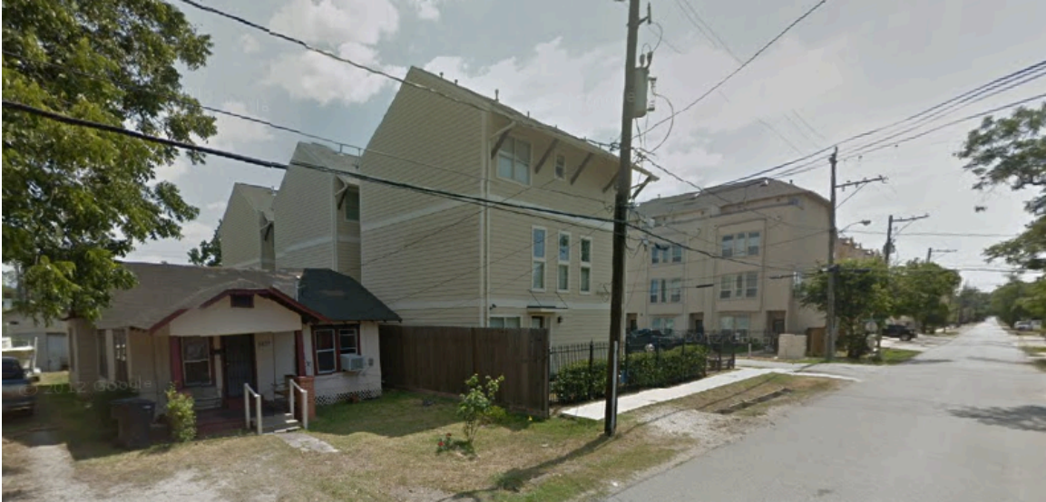
FIGURE 13: Redevelopment in the Cottage Grove neighborhood (Google Maps, 2014).
