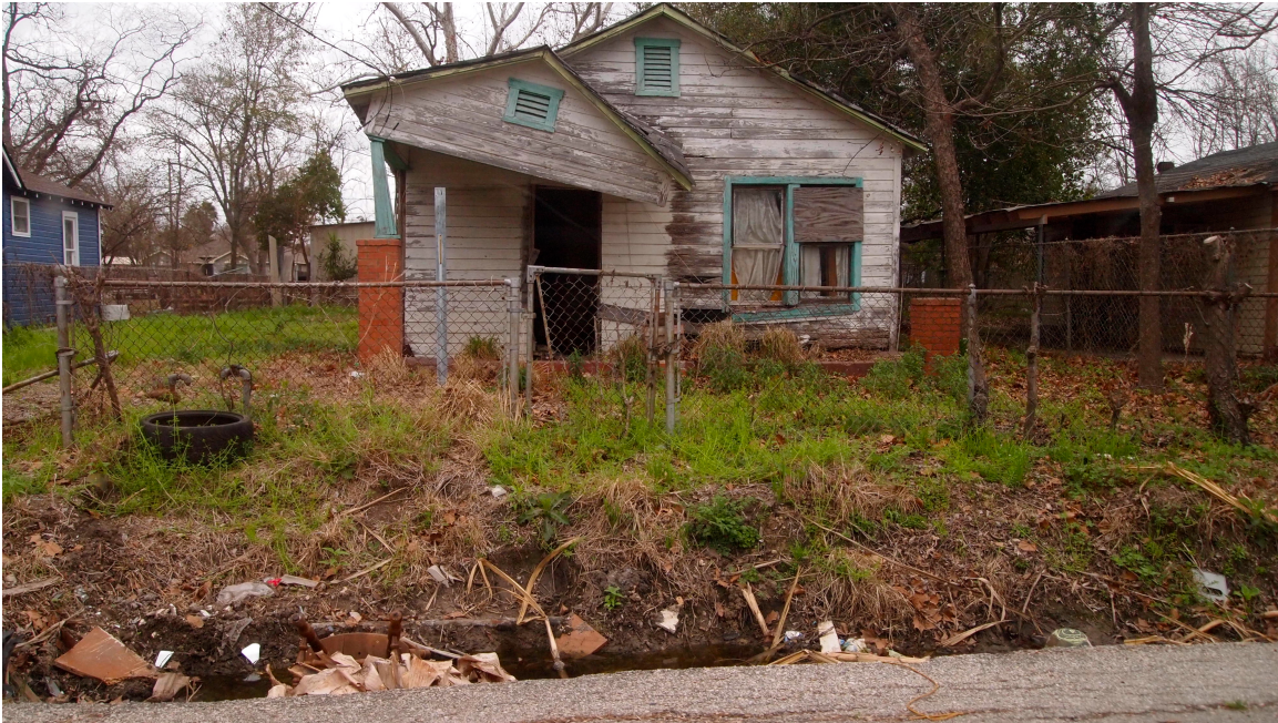
FIGURE 12: A roadside drainage ditch in the Fifth Ward filled with flow blocking debris.
