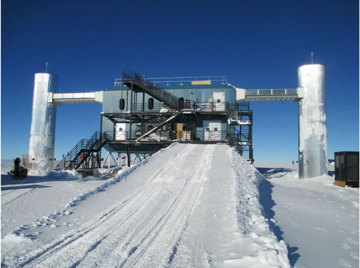
**Figure 23:** The IceCube Laboratory at South Pole. DOMHub computers located within the ICL communicate with all DOMs on a respective string. The cables carrying power and information for each DOM arrive at the ICL and enter the building from either the left or right tower near the ceiling (Photo credit: J. Daughhetee).
