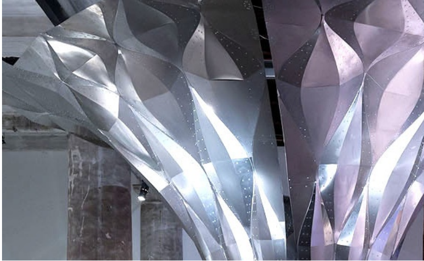
Figure 3.3: The “Arum” surface was designed by Zaha Hadid Architects in cooperation with Robofold for the 2012 Venice Biennale. The “peddles” are manufactured by folding metal sheets along curved creases by robots.
