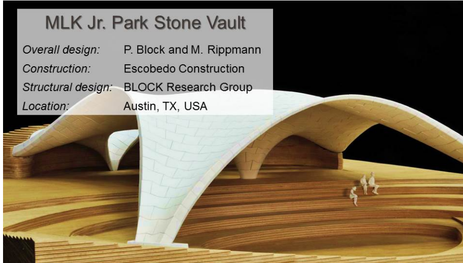
Figure 2.2: This masonry structure designed by P. Block is going to be constructed in Austin with local Texas limestone. It is self-supporting, as it can support its own weight with compression force only without reinforcement.
