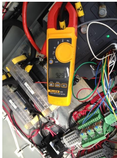
Figure 44. Torque-voltage slope identification using a clamp ammeter
