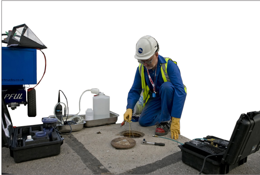
Fig 16: Image of worker checking ground water level at monitoring well.
