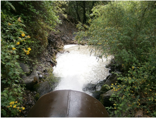
a. Uvas Reservoir Outlet into Uvas Creek.
