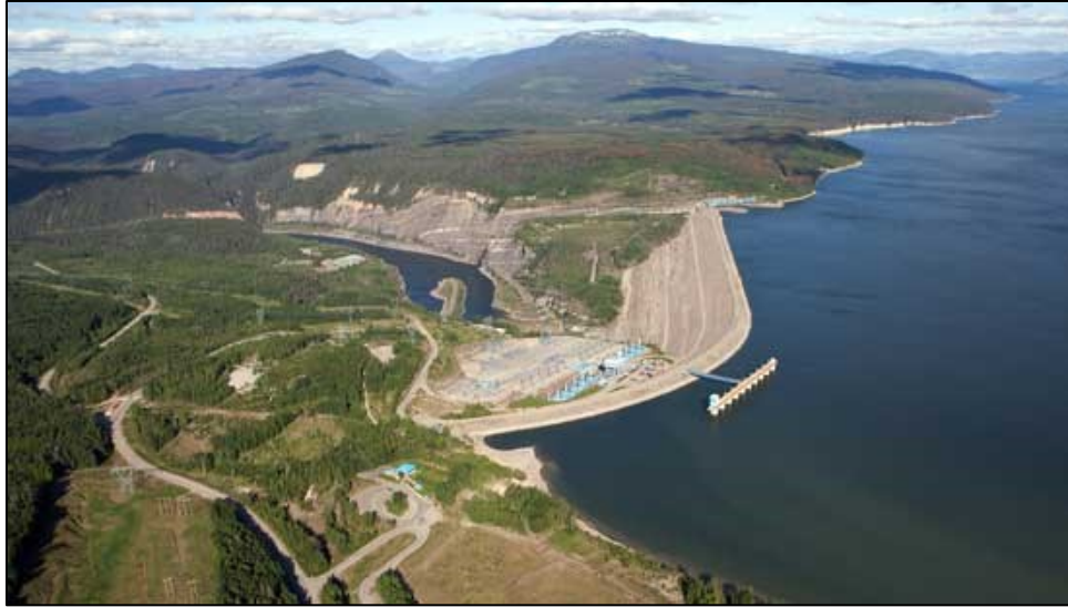
Figure 5.9 W.A.C. Bennett Embankment Dam, showing orientation of dam, spillway, and G.M. Shrum Generating Station (energeticcity.ca).
