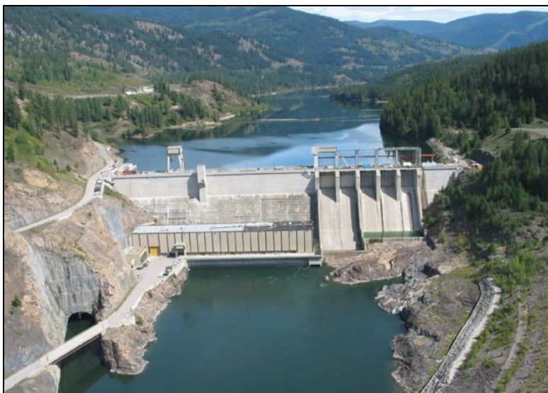
Figure 5.5 Seven Mile Dam – photograph of upstream view of the concrete gravity structure.
