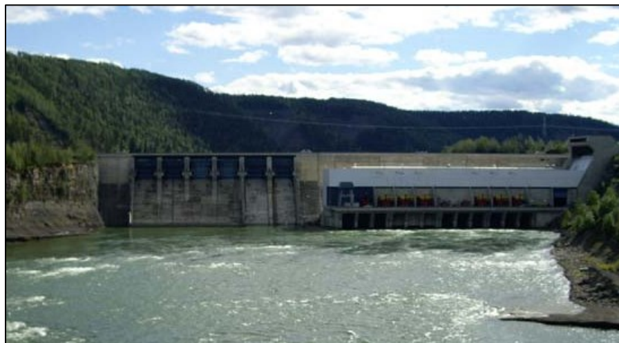
Figure 5.2 Peace Canyon Dam, showing the six-gated overflow spillway on the left (river right) and the powerhouse on the right (river left).
