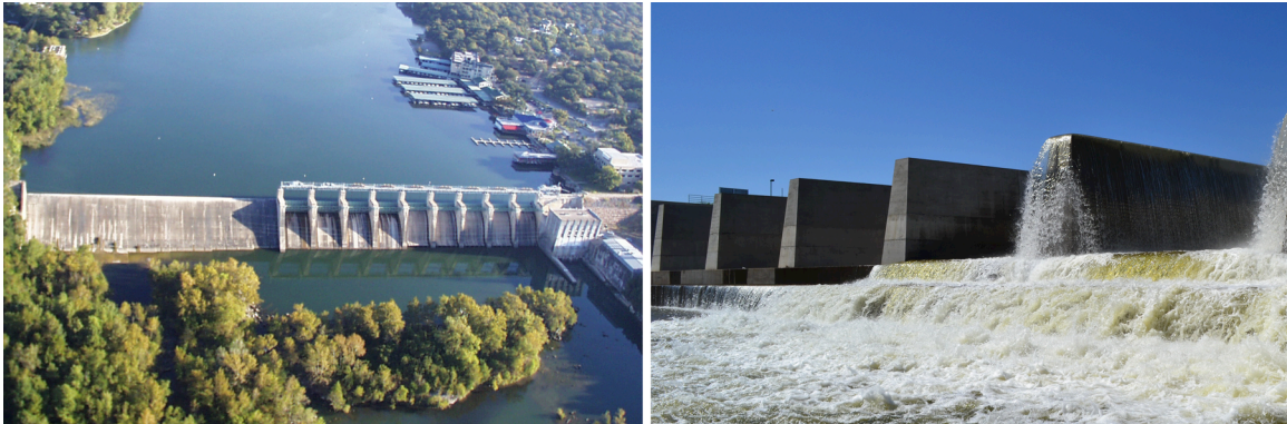
Fig. 21. Photos of staged ogee-crested weir (Tom Miller Dam, TX) and staged labyrinth weir (Lake Townsend, NC). Courtesy of: Michael Johnson and Brian Crookston
