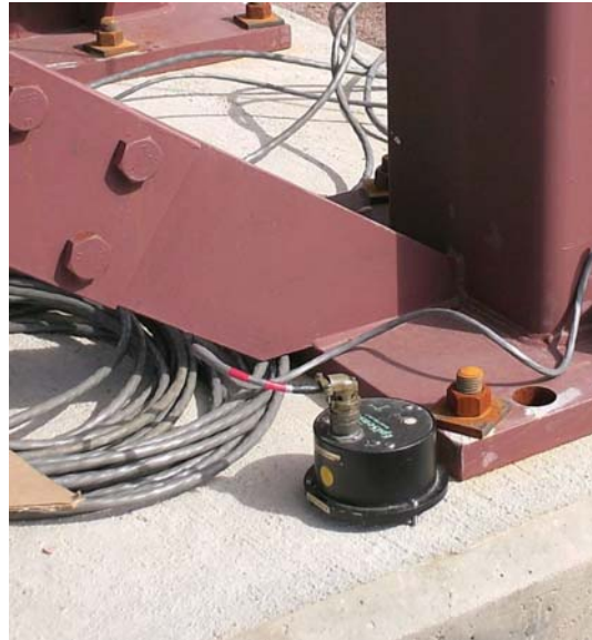
FIGURE 3.3. (From Star 2011) Location of installed triaxial accelerometer on the test structure.
