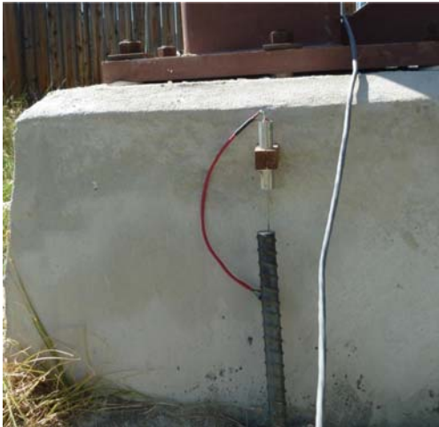
FIGURE 3.4. (From Star 2011) Picture of LVDT installed on corner of foundation slab.
