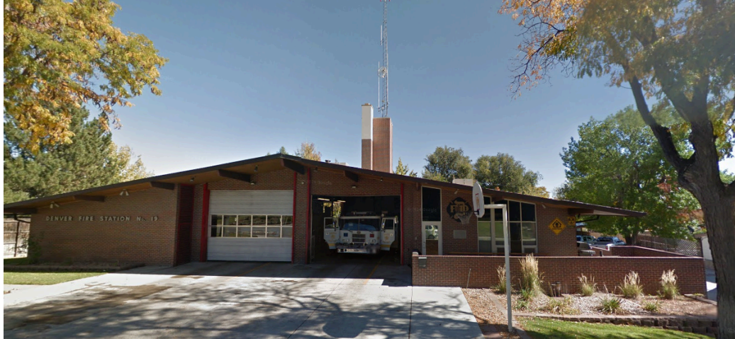
Figure 16. Typical brick veneer construction. Denver Fire Station #19. 137
