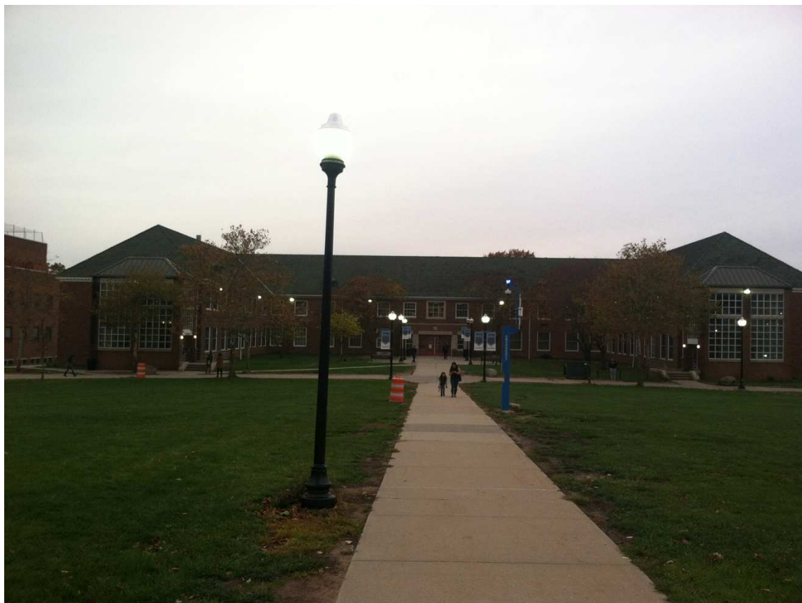
Figure 7: Willowbrook Building 19 East Side. Photo taken by Michael Ely. November 23, 2014.
