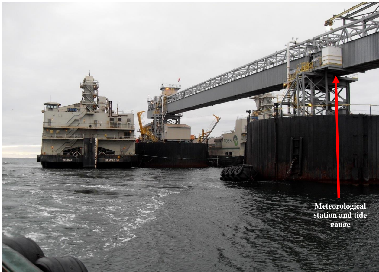
Figure 2. Red Dog Port Facility lightering dock and conveyor. Both of the 5000t lightering barges are visible, docked at the end of the conveyor facility. Photo by David Atkinson 2006.
