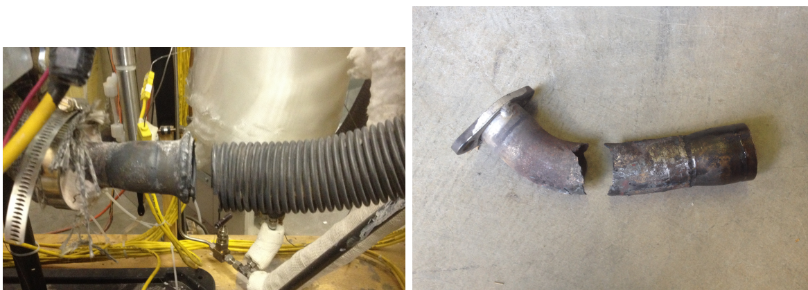
Figure 3.14: Two examples of exhaust line failure
