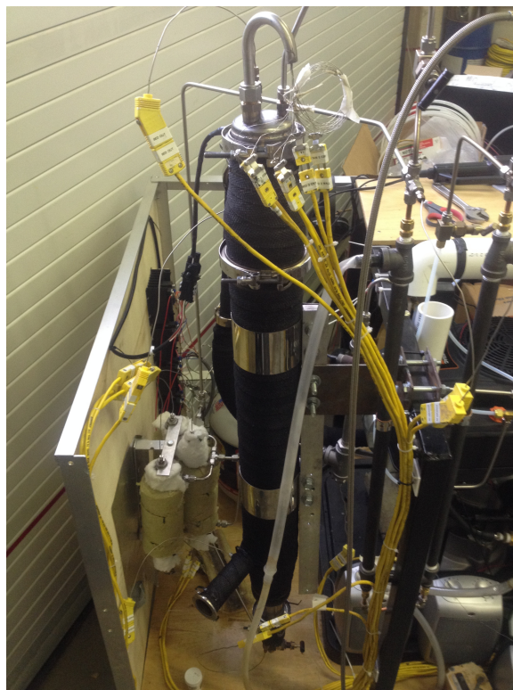
Figure 3.4: Installed steam reformer, shown with thermocouples and inner thermal wrap insulation
