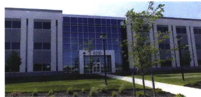
Figure 31. The Entrance at 6210 Guardian Gateway (Source: St. John Properties)
