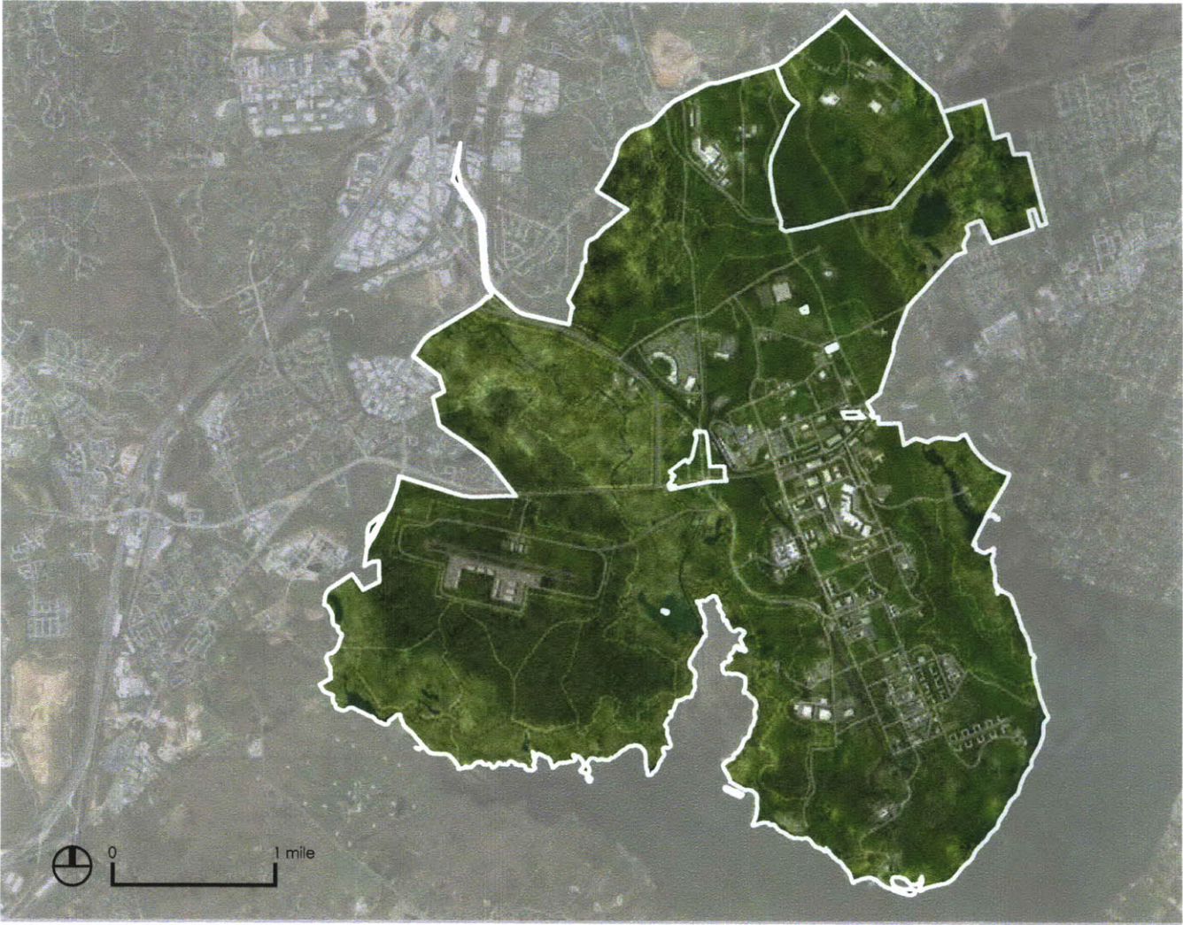
Figure 79. Site Plan. Rendered site plan of the design proposal. (Source: Fort Belvoir DPW)
