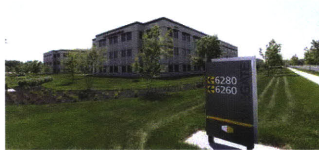
Figure 30. 3 Story Office at the GATE (Source: St. John Properties)
