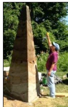
Spraying to slow the cure
