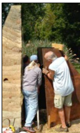
Setting the steel
