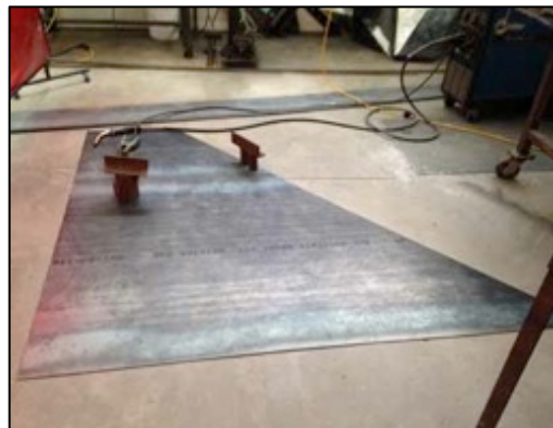
Welding the pieces together
