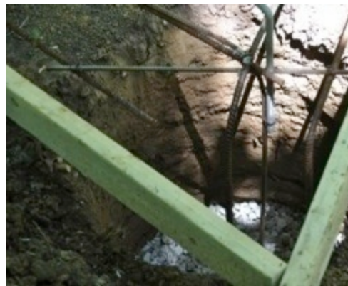
Steel Reinforced Piers
