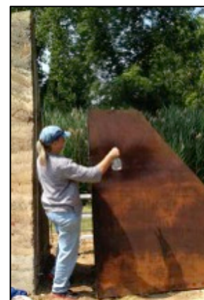
Acid spray to remove marks
