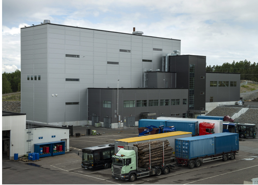
Figure 1.1: The CD7 building at Scania Technical Centre (STC) with preparation halls and support offices.
