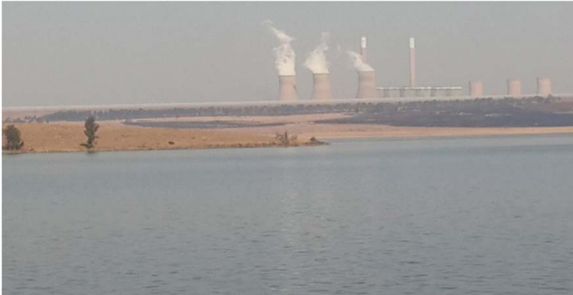
Figure 1.2: Witbank dam showing the proximity of the coal power station
