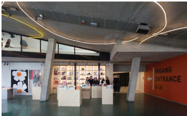
Figure 10.15 ~ Kunsthal slanted columns.jpg Kunsthal Rotterdam. Photo indicating the slanted columns in response to the ramped floor above. Source: OMA
