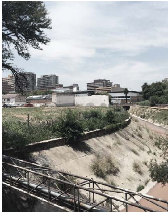
Figure 3.8 ~ Apies river channel.jpg Source: Author
