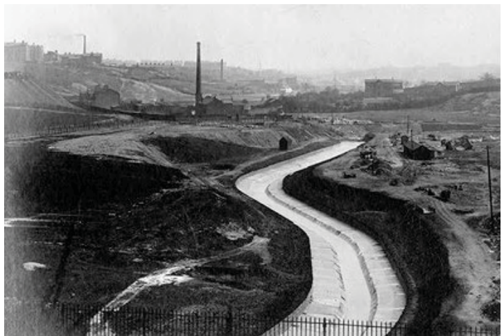
Figure 3.5 ~ Culverted River - controlled infrastructure.png
