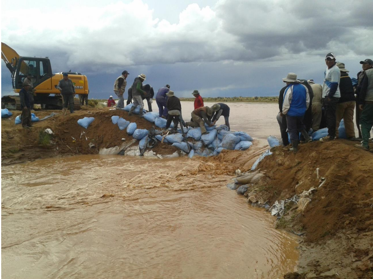
Figure 7: Irrigators work to dam the main canal.
