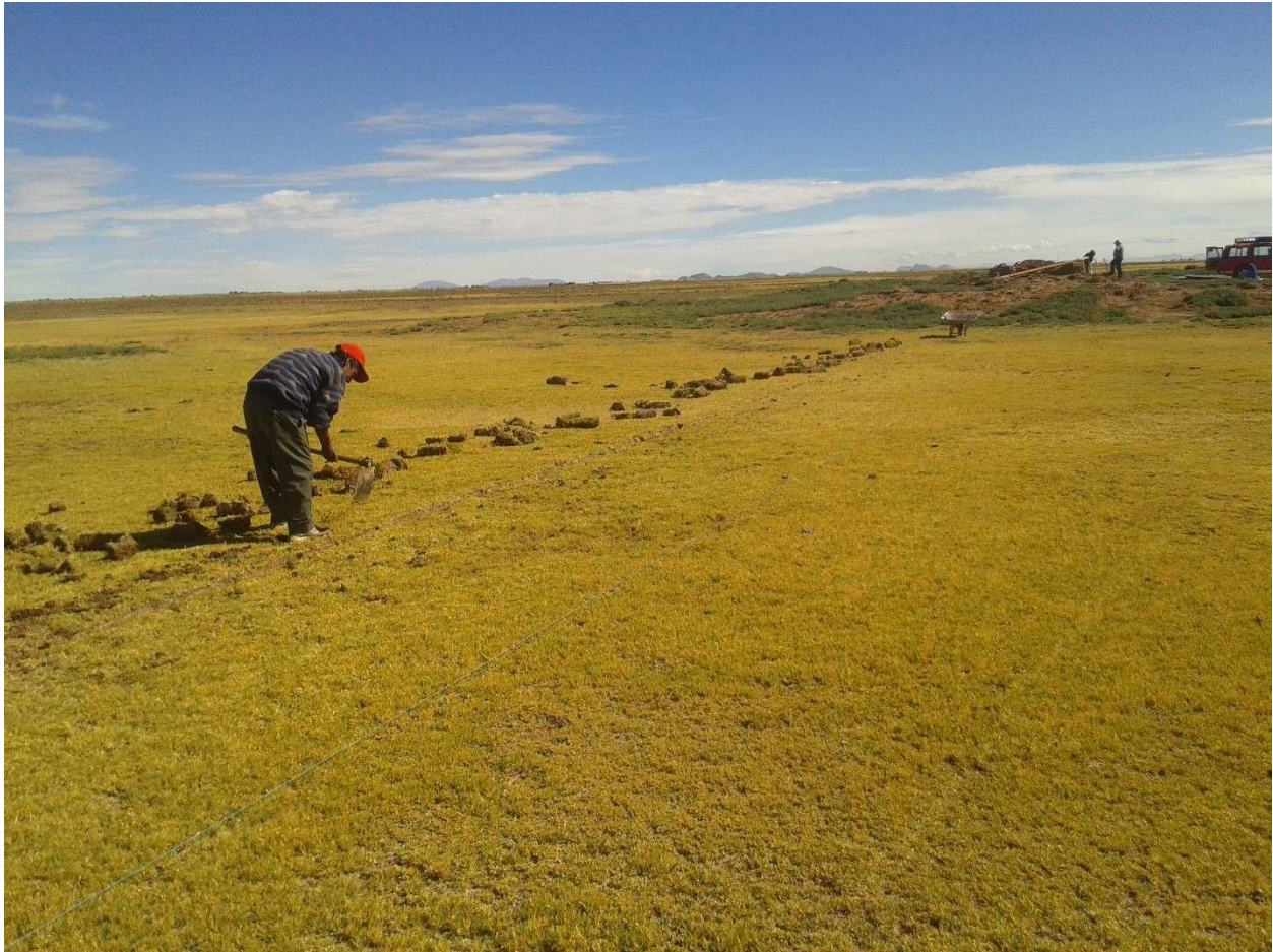
Figure 13: Severo preparing the ground to cut out tepes.
