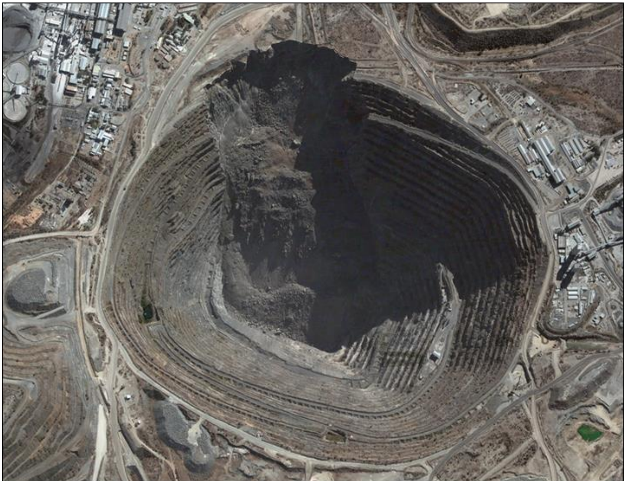
Figure 1.2. Quickbird image of 2004 North wall failure at Palabora. Note the proximity of access shafts to the crest of the East wall to the right of the image.
