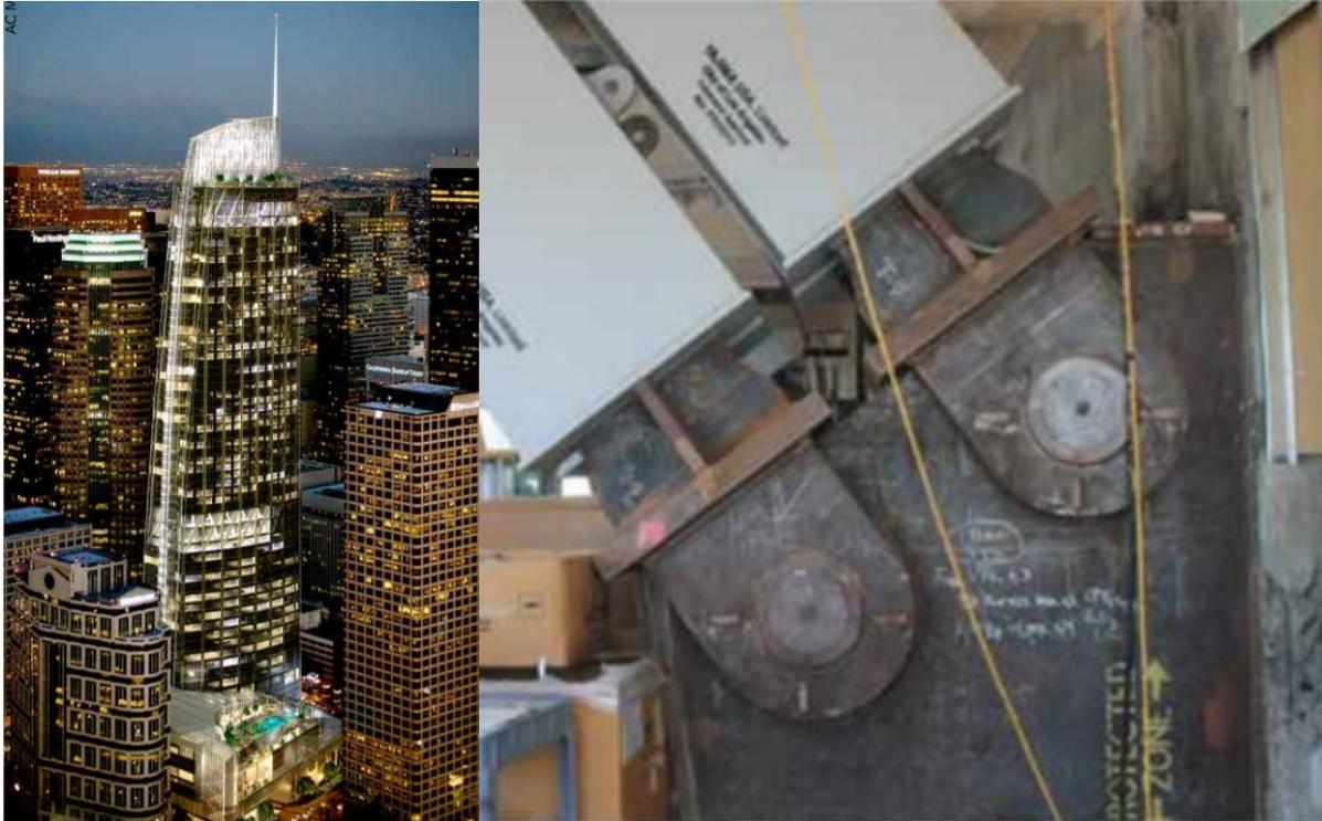
**Figure 5: Wilshire Grand (a) location in downtown LA (b) outrigger connection to core wall (Nieblas, 2017)**
