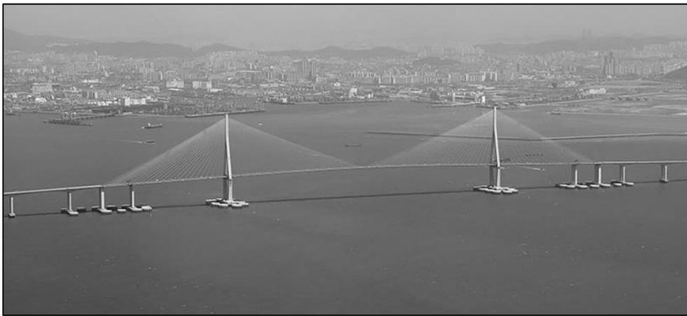
Figure 6.11: The Incheon Bridge, South Korea (Single Intermediate Pier)
