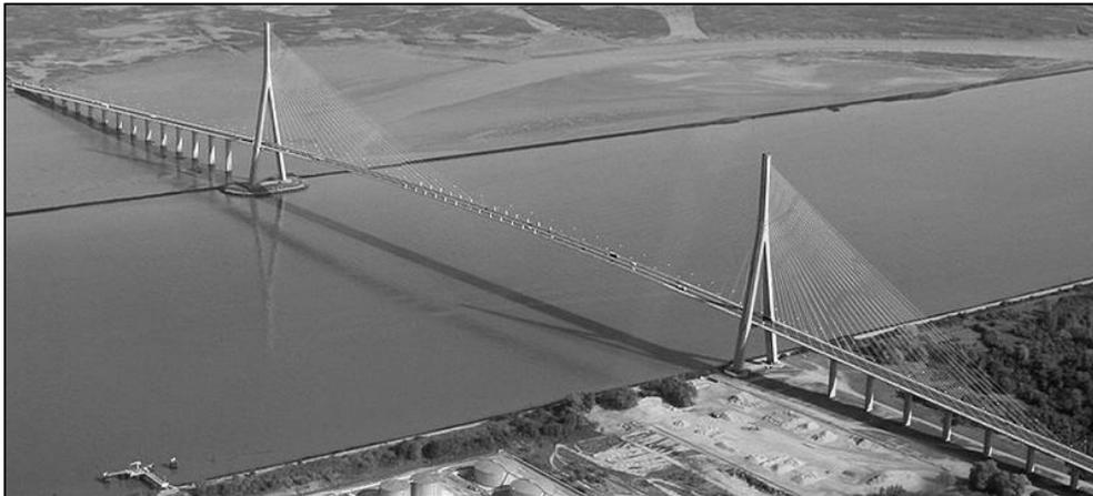
Figure 6.12: The Pont de Normandie, France (Multiple Intermediate Piers)
