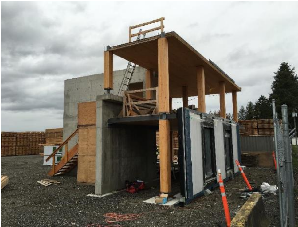
Figure 3-10 View of the mockup with one type of prefabricated panel
