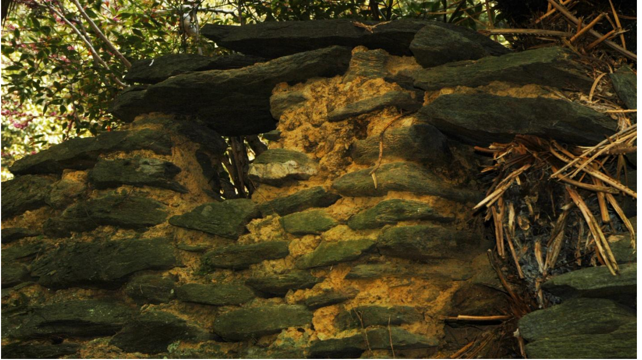
Figure 4-1. Detail of tuff bricks of the Kozasa Fortress, influenced by Korean architectural techniques
