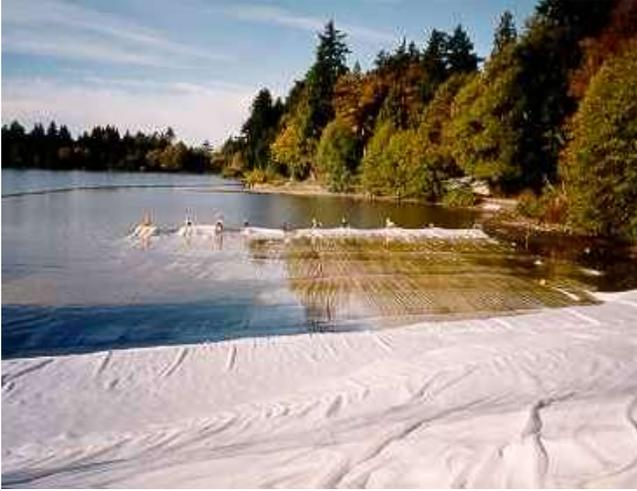
Figure 5. Laying of Silt Curtain
