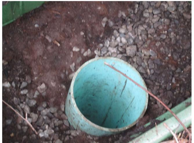
Figure 25. Access Point for the Wetland Outlet Control Valve System
