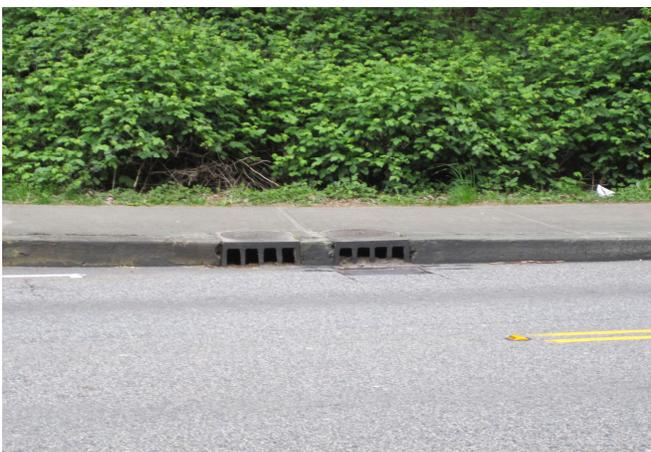
Figure 17. Storm Sewer on the Stanley Park Causeway
