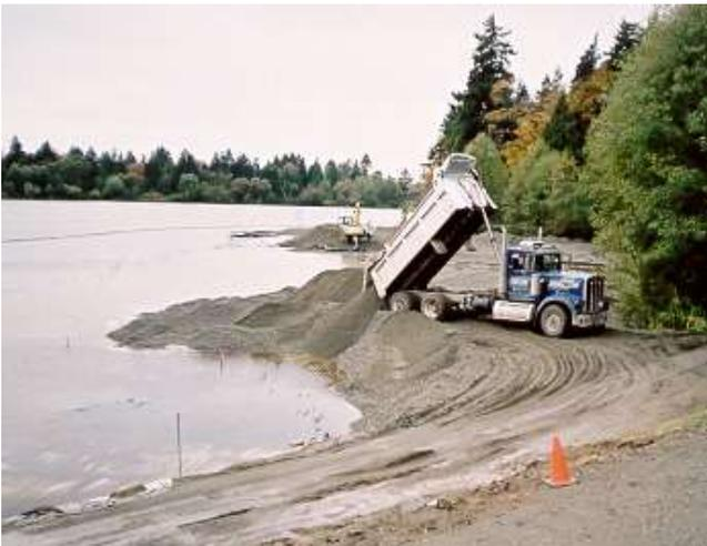
Figure 6. Construction of the Berm
