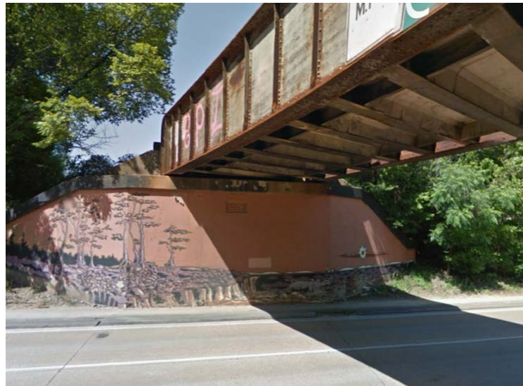
Figure 11: Dallas Drive Underpass current mural (Google Maps)
