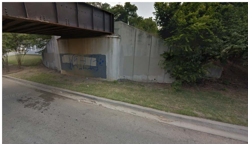
Figure 7: Underpass at Robertson and Bell
