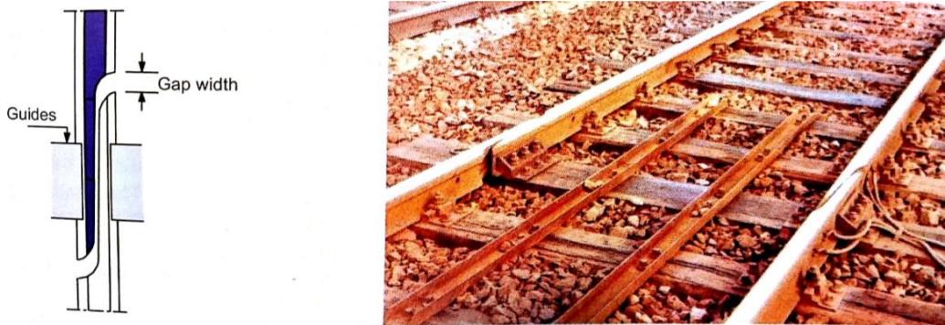
Figure 2.12 Expansion joint, (Esveld, 2001).
