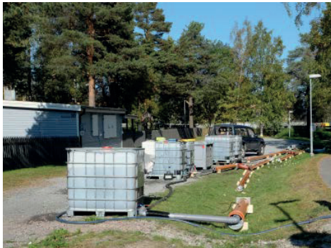
Figure 2. Swale water supply system comprising IBC tanks, longitudinal inflow pipe, and two lateral inflow distributors.
