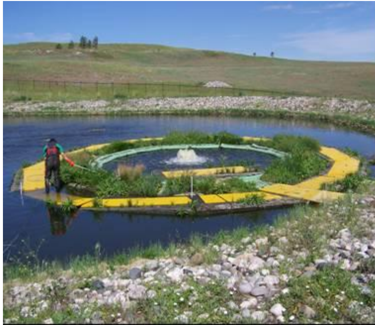
Figure A.1. A 232 m 2 FTW in an aerated lagoon at Rehberg Ranch Subdivision, Billings, MT USA. The FTW is circular, with a radial fountain pump installed in the center. The body of the island is designed to float below the surface in order to maximize constituent uptake by biofilms growing on the plastic matrix. Parameters being tracked include suspended solids, BOD, nitrogen and phosphorus. The island was installed by Headwaters Floating Island, LLC during November 2009, and planted during the spring of 2010. Periodic water quality testing is being provided by the City of Billings, MT and Floating Island International, LLC.
