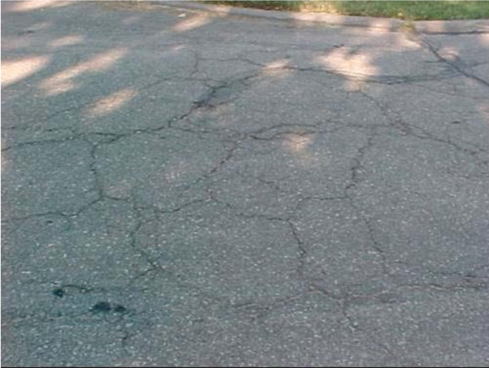
**Figure 2.3 Fatigue Cracks on Asphalt Pavement**
