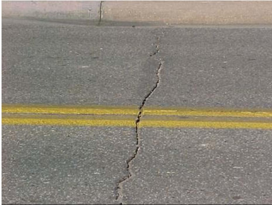
**Figure 2.4 Low-Temperature Crack on Flexible Pavement**
