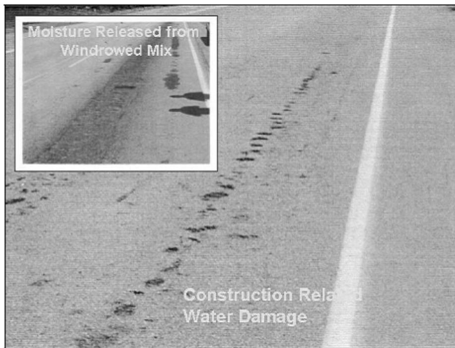
**Figure 2.6 Typical Localized Failure Due to Moisture Damage (Hicks et al. 2003)**
