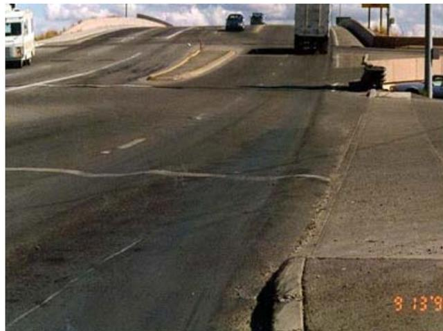
**Figure 2.1 Rutting in the Wheel Paths**
