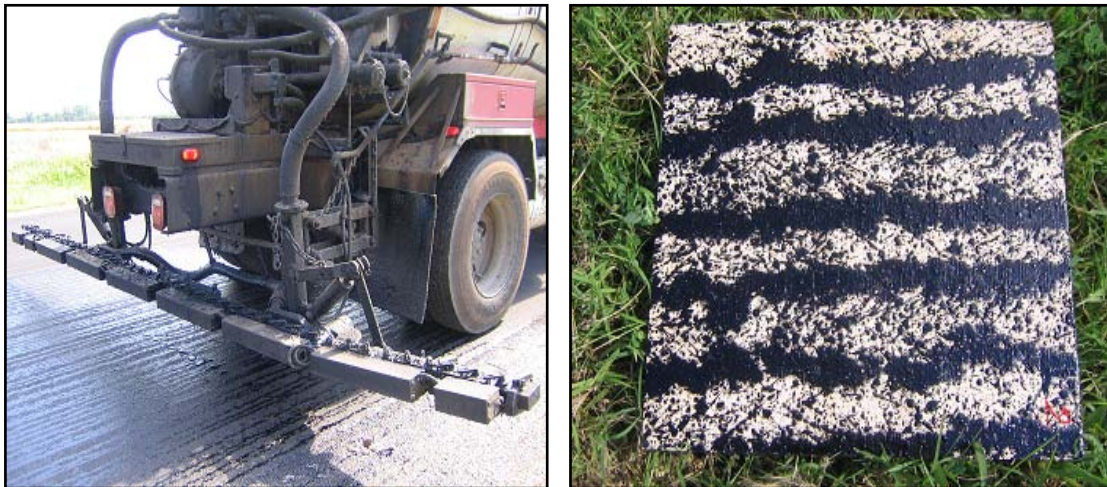
Figure 3.4 Tack coat application and measurement on US-160
