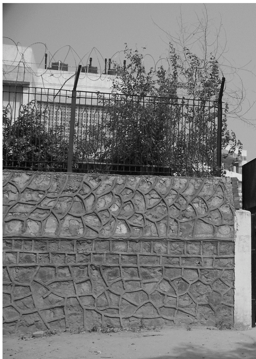
Figure 2 The front wall of Government Hindi
