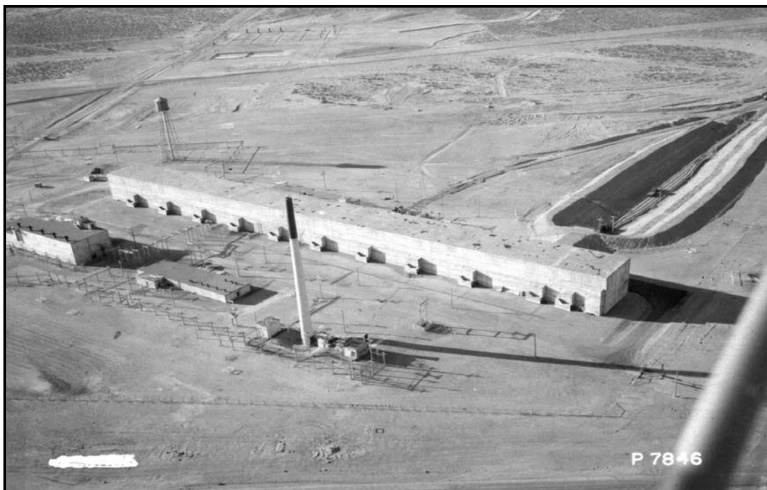
Figure 20. Hanford Engineer Works, Plant T (221-T, “Queen Mary” Separation Plant), 1944. Hanford Declassified Document Retrieval System. No. N1D0030560.
