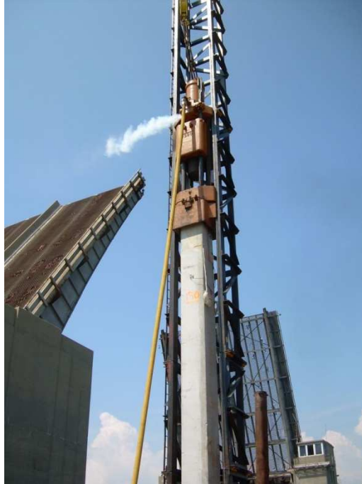
Figure 1.1 Installation of a precast concrete pile by an air hammer.
