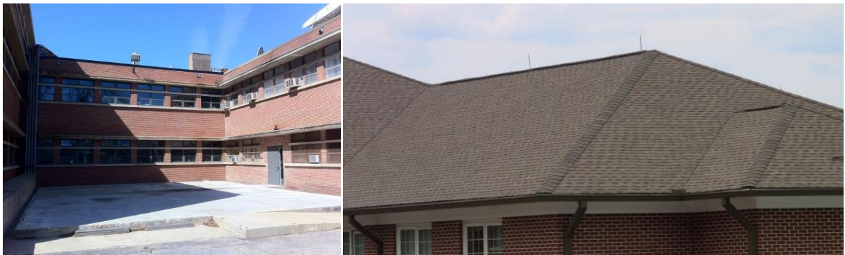
Figure 3.7: A building façade and a residential roof structure
